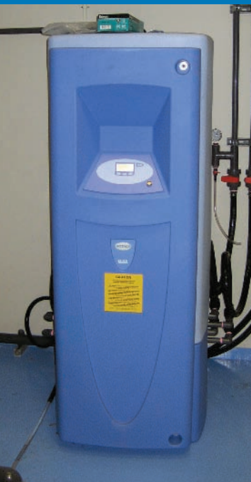
◀ A modular central water system for a small research, clinical or pharmaceutical laboratory, featuring a small foot print, 3 to 12 points of use, a couple of chemistry analyzers and Type II or USP quality water.
